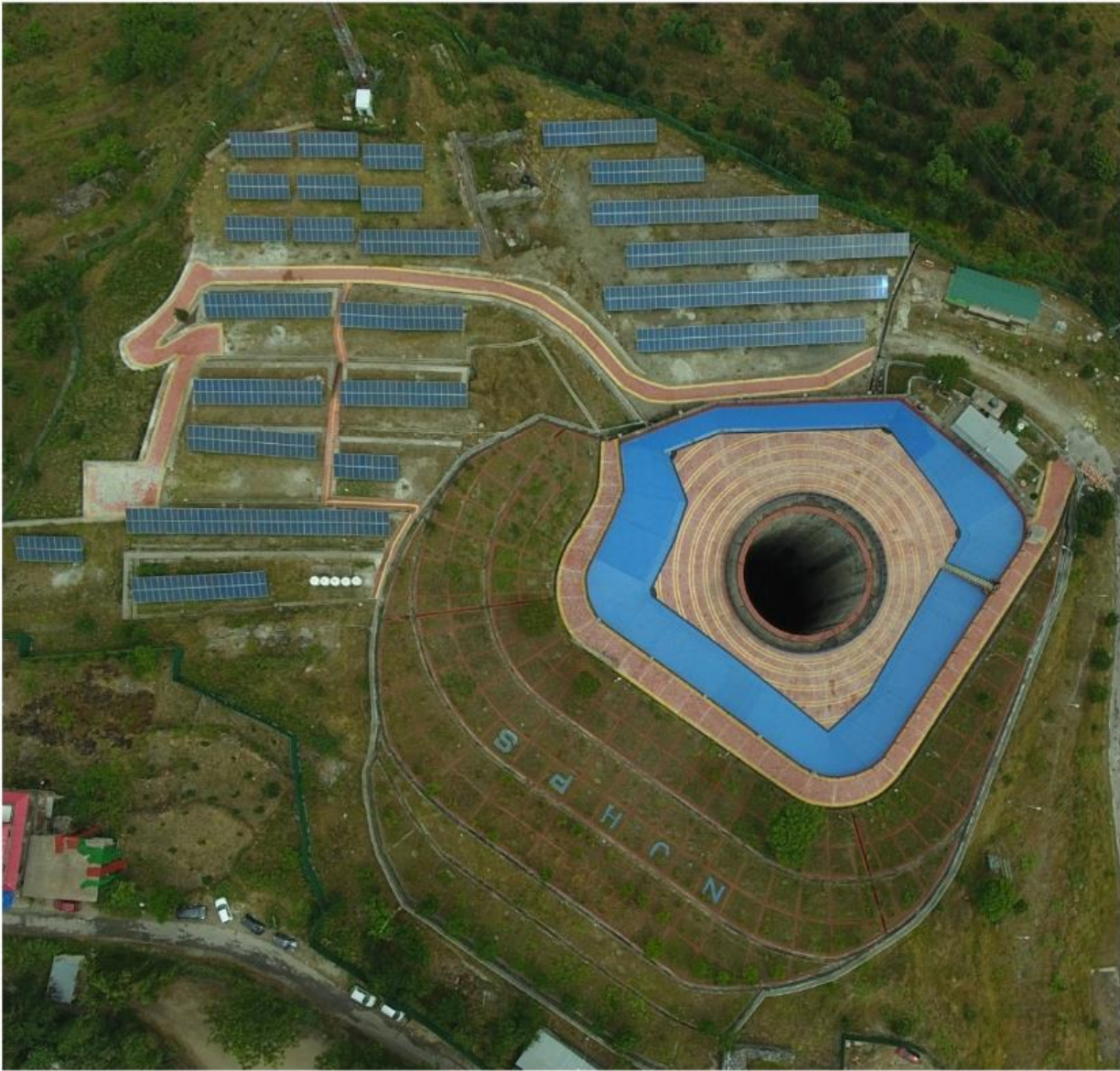
301 Meter Deep Surgeshaft of Nathpa Jhakri Hydro Power Station, Jhakri (HP)
