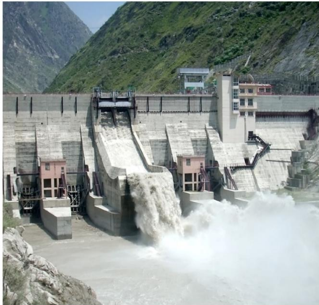
Dam Site of 1500 MW Nathpa Jhakri Hydro Power Station, Nathpa (HP)
